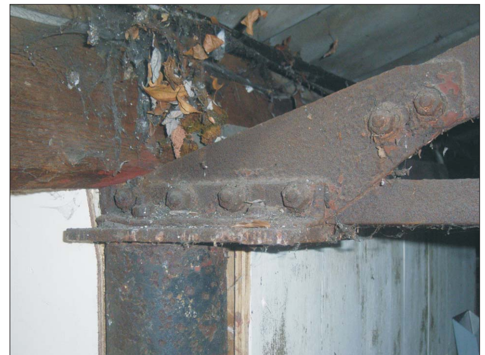
Plate 15: Building C - Interior. Roof truss resting on cast iron column showing cut back edges
