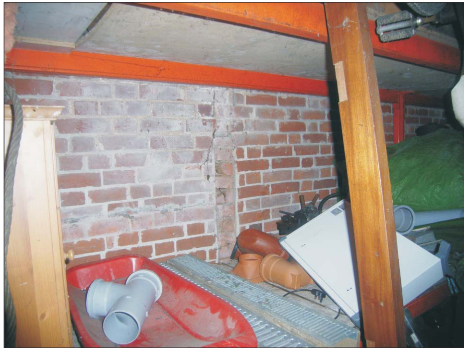
Plate 16: Building C - Interior. Evidence of removed partition
