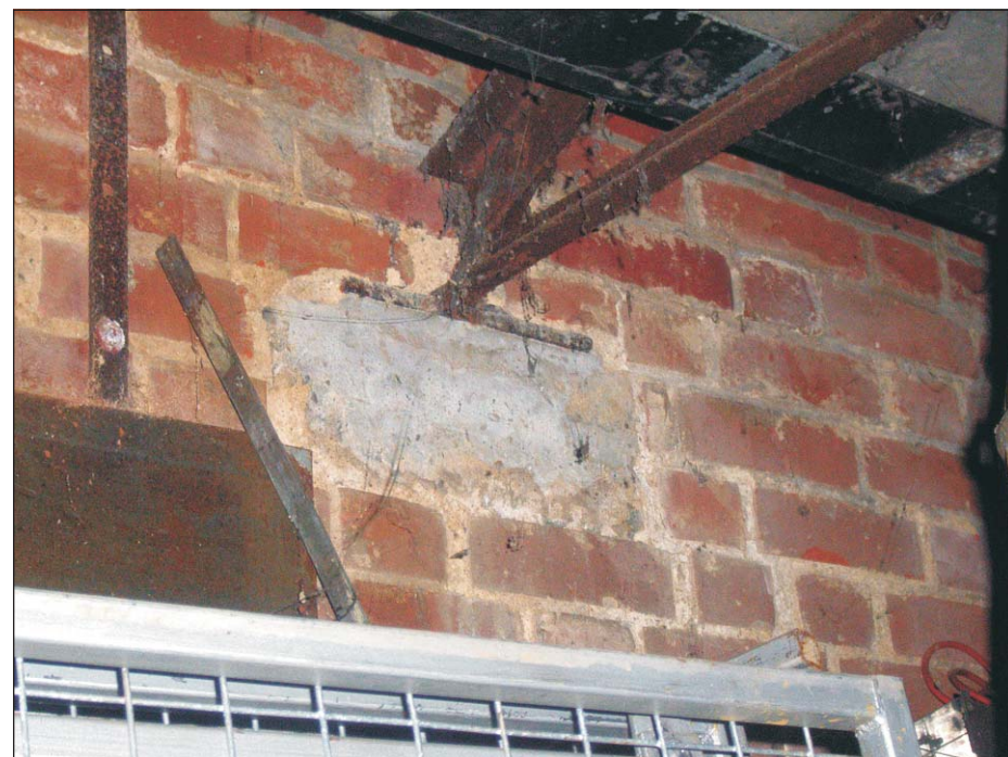
Plate 14: Building C - Interior. Rooftruss resting on padstone in north wall
